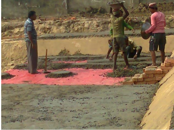
Concrete work on December 31, 2010
