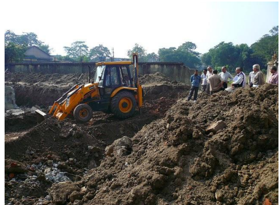
Construction site on December 11, 2010
