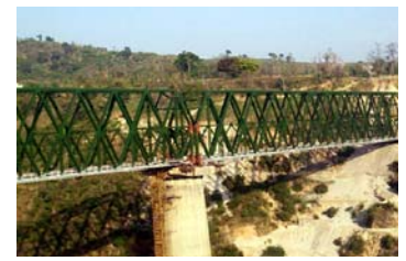
Supported at Pier launched towards Abutment
