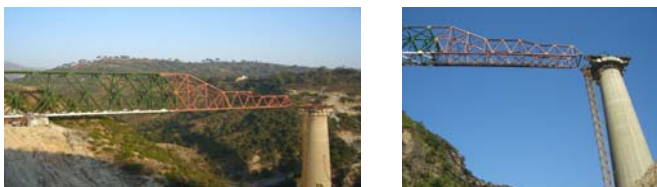
A stage in launching (Nosing marked in red)
