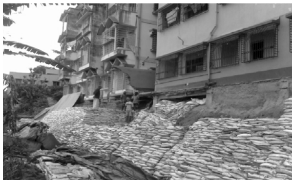
Both River Palace & Ganges Valley Apartments badly affected, some protective sand bag dumping being undertaken by Flat Owners
