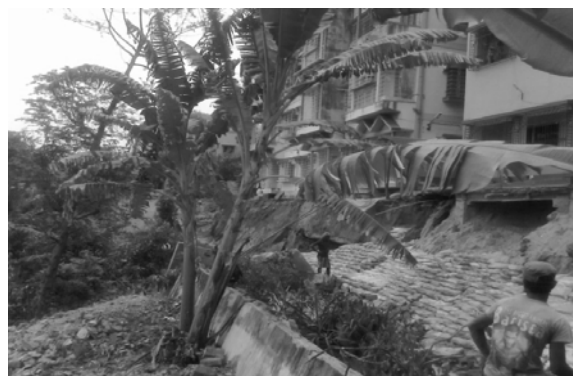
Filling material below Plinth of Both River Palace & Ganges Valley came out as a result of Erosion
