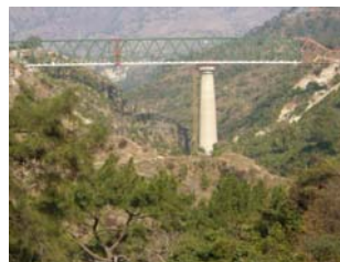
Truss reaching abutment at other end
