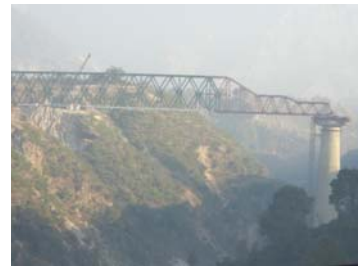
Truss supported by nosing at Pier
