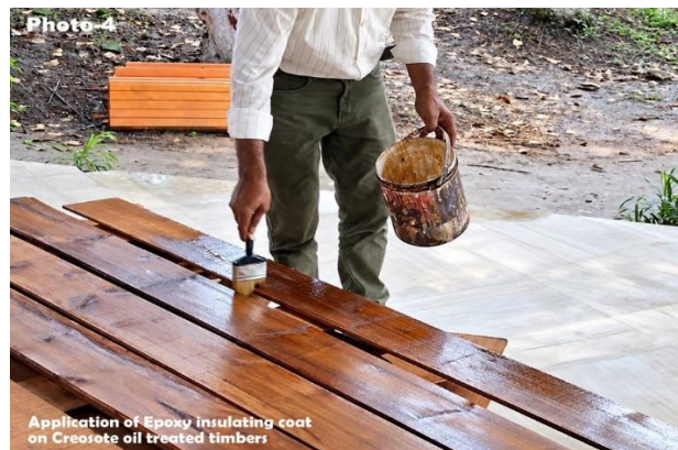
Photo-4 Application of Epoxy Insulation coat on creosote oil treated timbers
