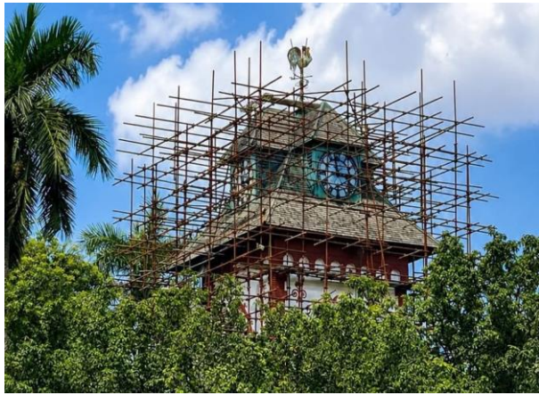
Photo-1 View before rehabilitation
