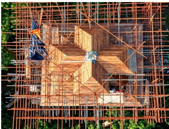
Photo-7 Installation of top layer timbers
