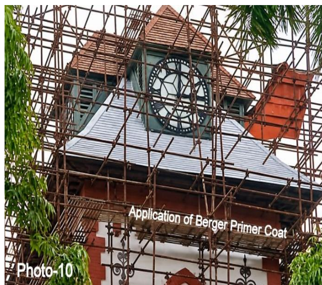
Photo-10 Application of Primer (undercoat)
