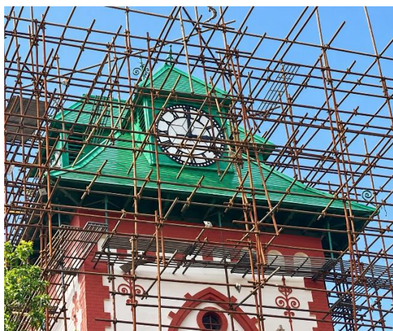
Photo-11 Application of Final Hi-Gloss Paint
