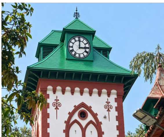
Photo-12 Completed View (Scaffoldings removed using AI)
