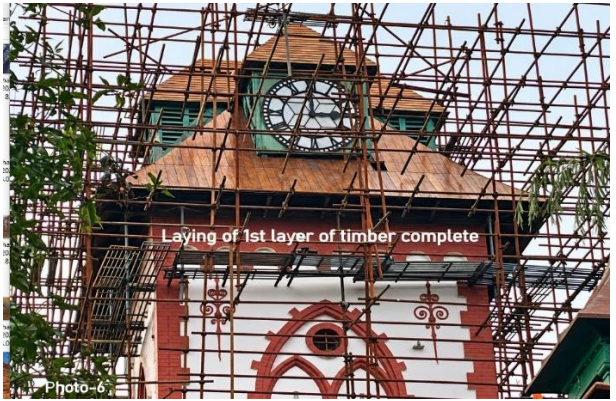
Photo-6 Completion of first layer timber fixing
