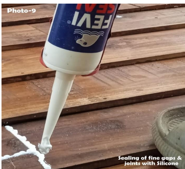
Photo-9 Sealing of fine gaps & joints with Silicone
