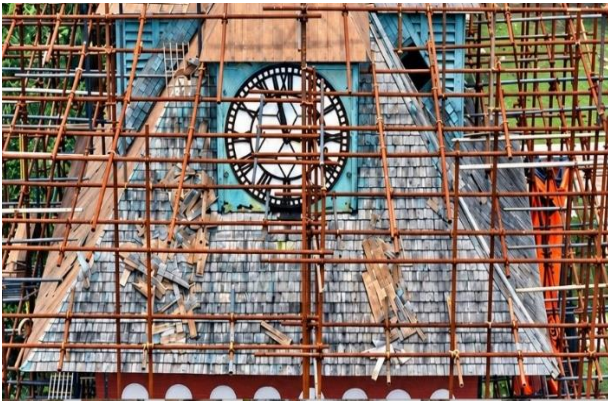
Photo-5 Entire top layer timbers being removed
