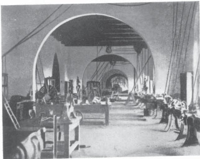
P.W.D. WORKSHOP, CONVERTED TO COLLEGE WORKSHOP
