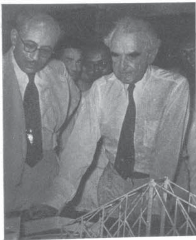
RICHARD NEUTRA, AN ARCHITECT OF INTERNATIONAL FAME AND JOSSEPH ALLEN STEIN, HEAD OF THE ARCHITECTURE, TOWN AND REGIONAL PLANNING DEPARTMENT INSPECTING THE MODEL HOWRAH BRIDGE MADE BY THE ARCHITECTURAL STUDENTS
